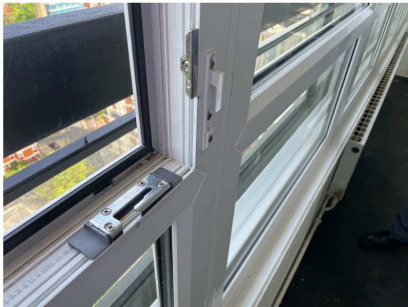
8. Hinge and fenestration details
